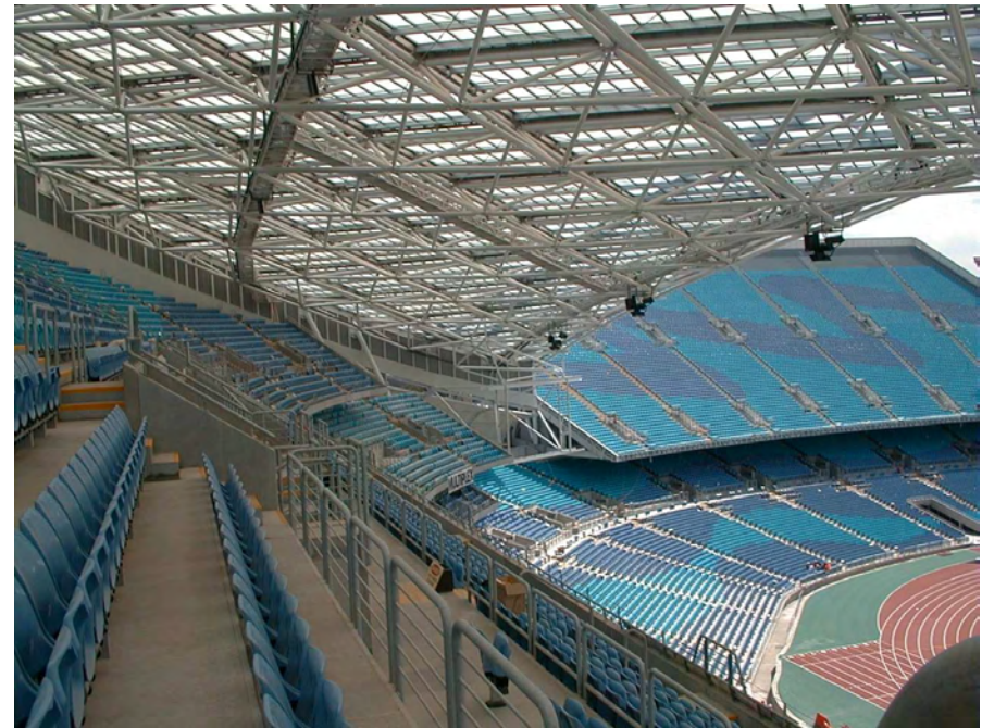
Optimum Daylight Transmission Roofing for Sydney Olympic Stadium
