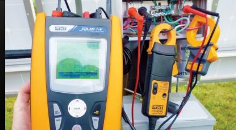
String Test & Commissioning
