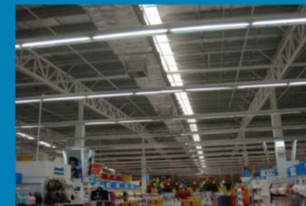
T5 Lamps Installation
