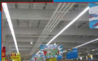
T5 Lamps Installation
