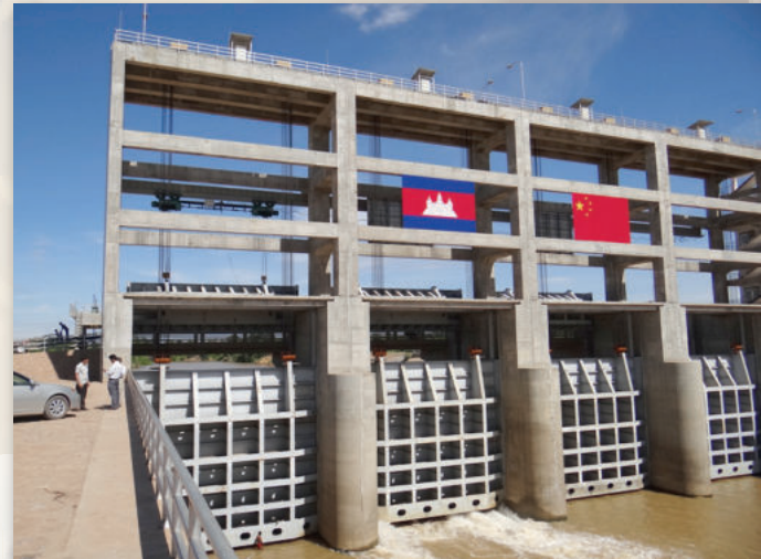
Flood Management System, Photo Credit: Try Thuon
